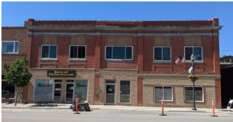
The original Courthouse/City Hall is a prime example of the Masonry Wall Massing, Detailing, and Punched Openings.
