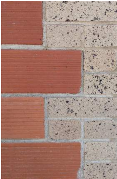
Example of Masonry Walls.
