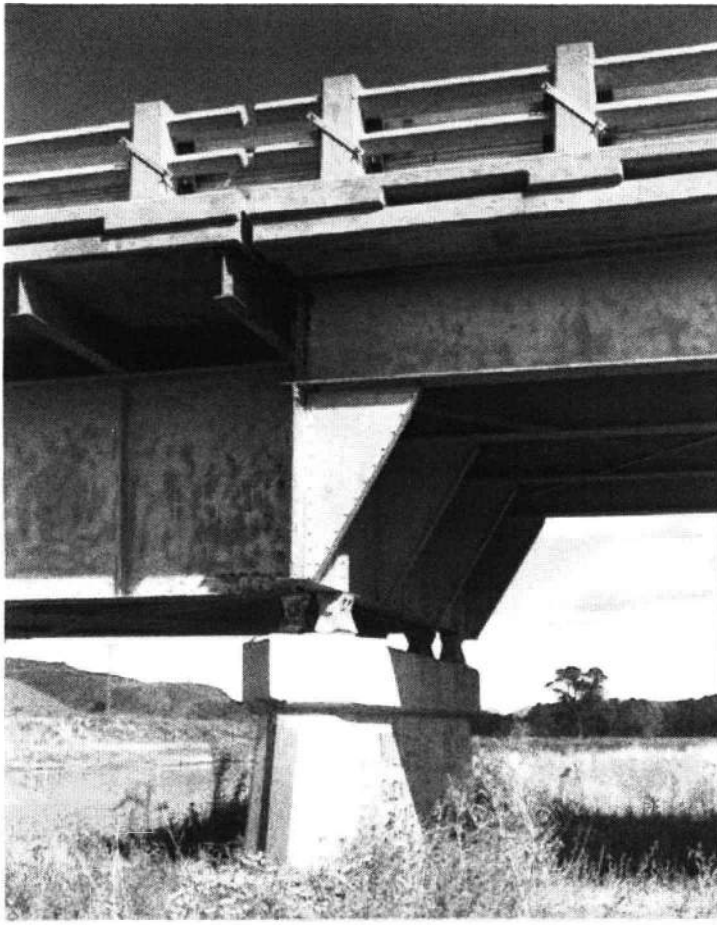
Photo 0003. Marias River Bridge. Detail. View to the east
