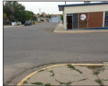
Figure 24 - Missing Curb Ramps
