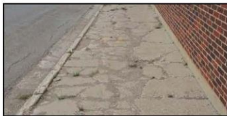
Figure 25 - Deteriorated Sidewalk
