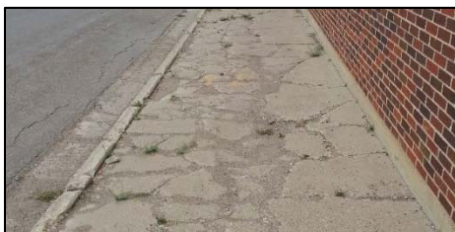
Figure 25 - Deteriorated Sidewalk
