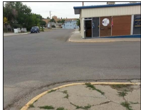
Figure 24 - Missing Curb Ramps
