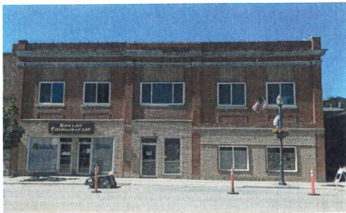
The original Courthouse/City Hall is a prime example of the Masonry Wall Massing, Detailing, and Punched Openings.
