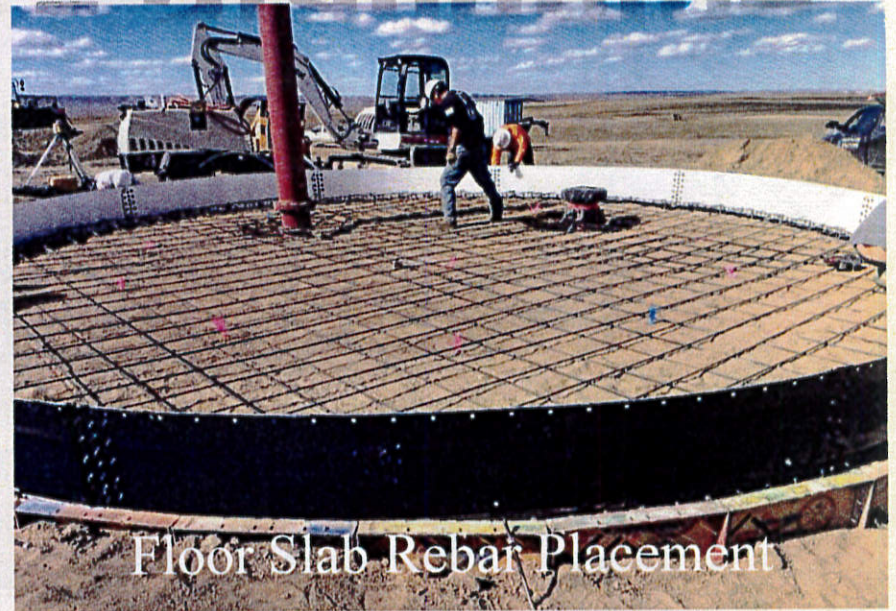
Standpipe Construction
