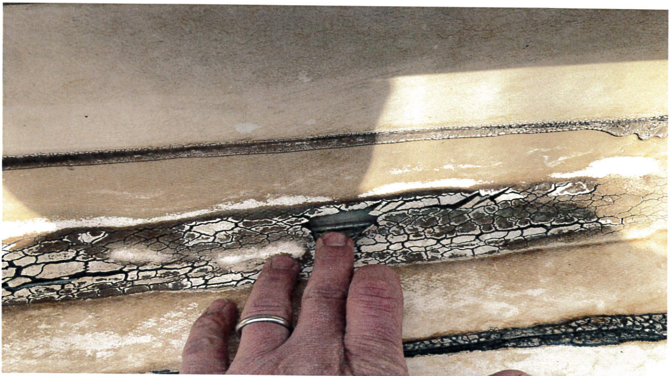
Damage to inside corner on second roof
