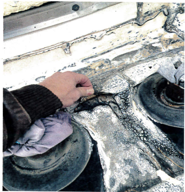
Damaged TPO on first roof
