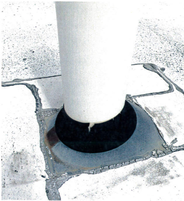
Roof boot damaged and needs to be replaced (There are 6 roof boots to replace)
