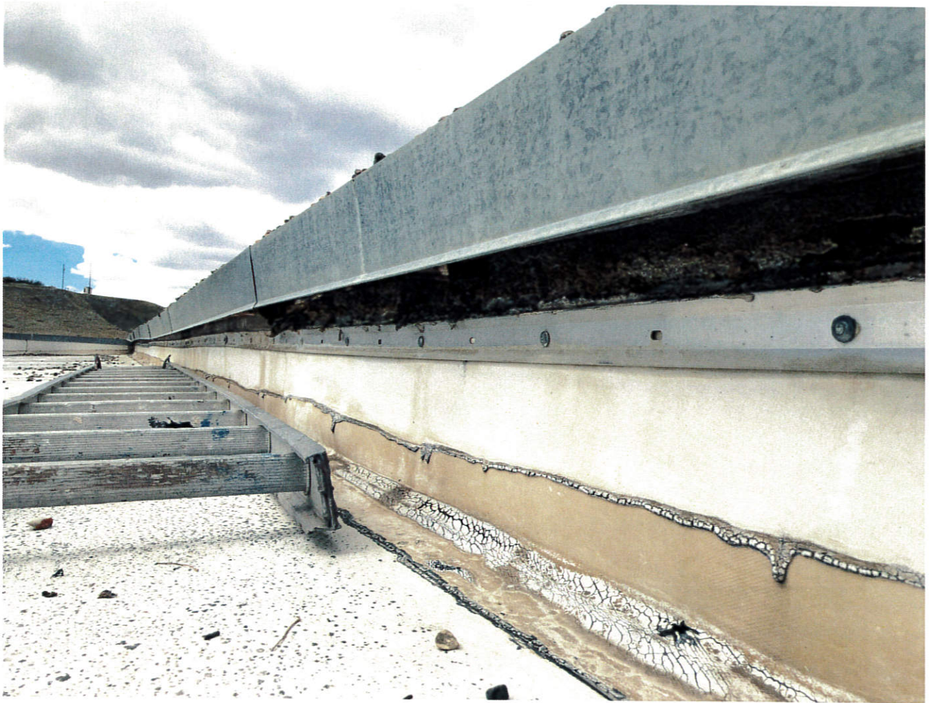
This is a picture of where the second TPO roof attaches to the main building and need to be repaired and coated
