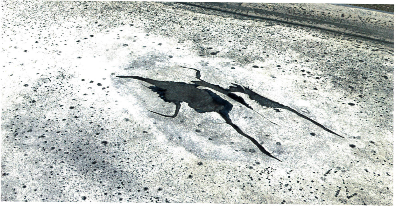
Picture of ripped and damaged TPO that must be repaired
